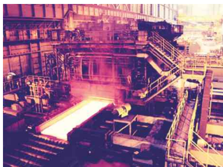
Slab Re-Rolling Mill
