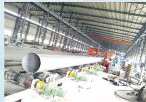
Stainless Steel Pipe Mill
