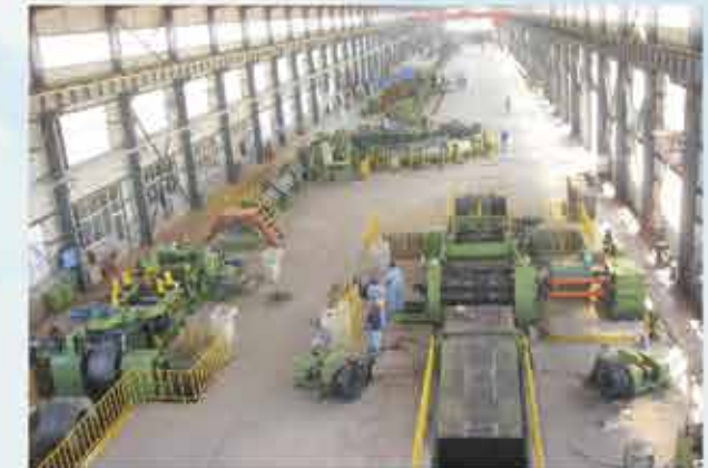
355mm ERW Pipe Mill
