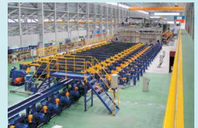
Chain Type Cooling Bed
