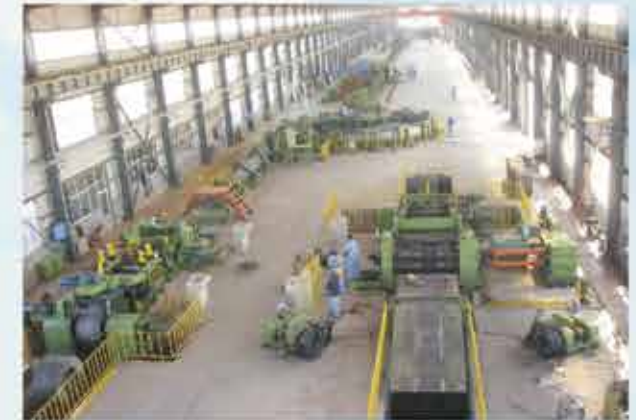
355mm ERW Pipe Mill
